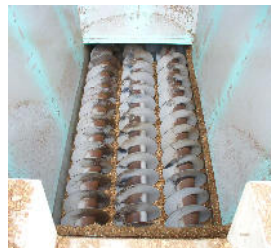
Mounting in discharge screw (wood-fired power plant)
